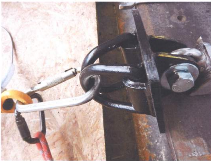
Fig. 7: anchor device type attachment eyelet, mounted at steel construction
